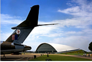
American Air Museum Duxford. Photograph with kind permission of Foster and Partners, all rights reserved width of the building entrance.
